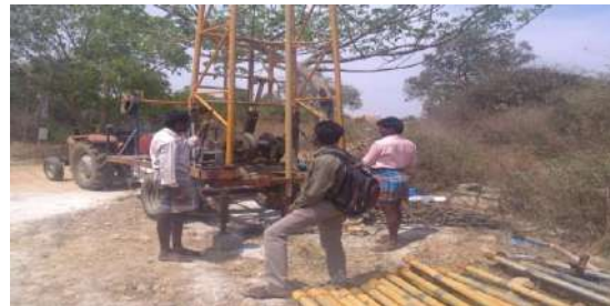
Repair works to control water wastage
